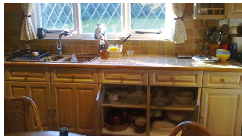
Figure 4 Fitted kitchen with plastic carcasses and removable doors
