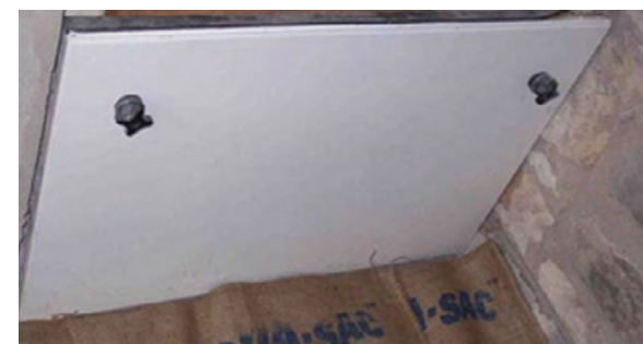
Figure 3 Door guard fitted to the internal door way
