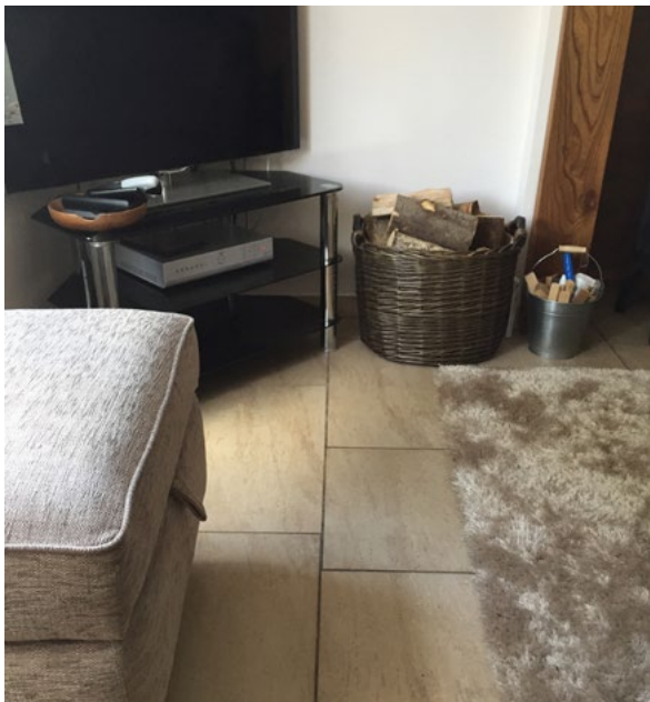
Figure 1 The ground floor is tiled throughout, using water resistant cement and grout – it can be hosed down and disinfected after a flood
