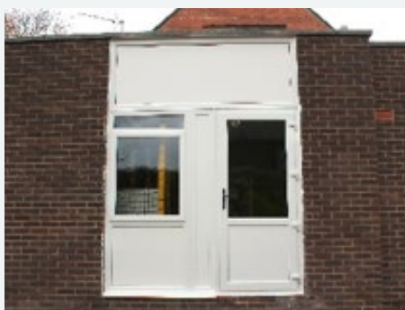
Figure 3 Flood resistant side door donated by www.floodsmartsystems.co.uk
