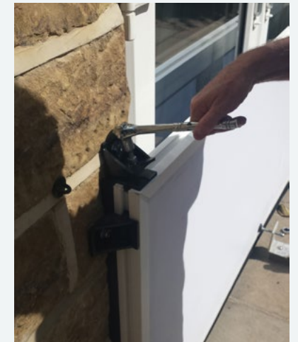
Figure 10 Fitting new (taller but light-weight) barriers
