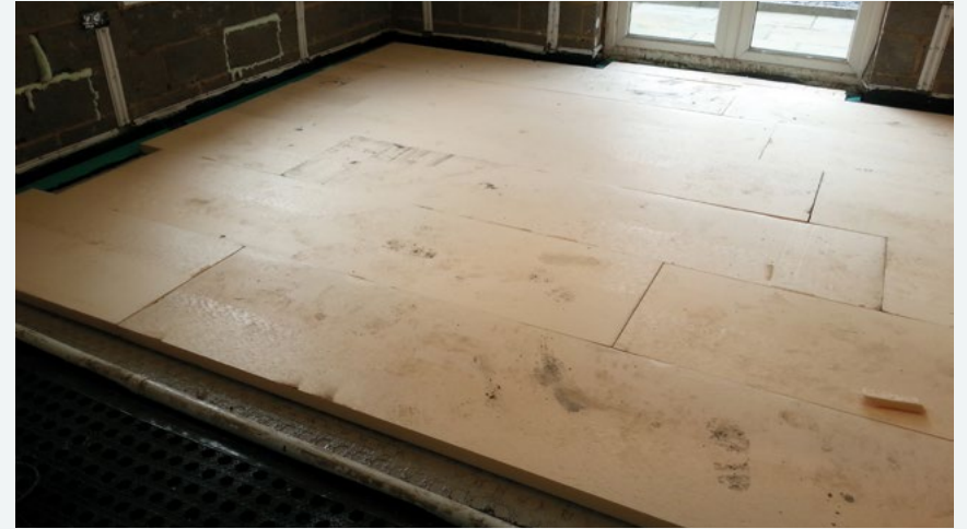
Figure 6 Closed cell (waterproof) insulation on the floor
