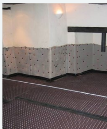
Figure 3 Internal walls now covered with a mesh membrane, and floors are covered with a studded membrane
