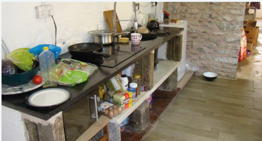
Figure 4 Granite topped kitchen shelving, with marble shelves and sandstone window mullions as a framework – some of the materials were found by the river, having been dumped there 18 months earlier!
