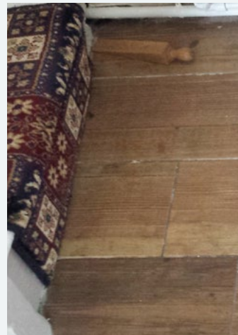
Figure 9 Wooden-floorboard-effect ceramic tiles in hallway and easily removable stair carpeting
