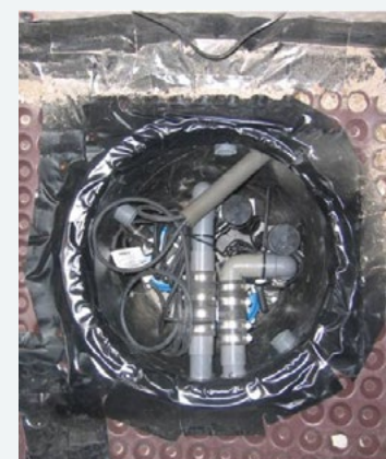
Figure 4 Two sumps (similar in size to a domestic dustbin) contain pumps designed to operate at different water depths.
