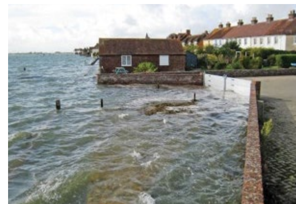
Figure 1 Flood barrier in action
