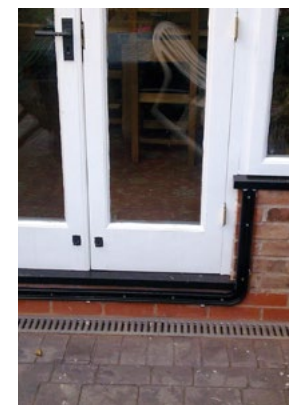
Figure 1 Non-standard doorway with unobtrusive barrier fittings
