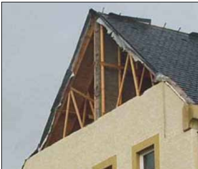
Fig 3.9: Gable wall failure
