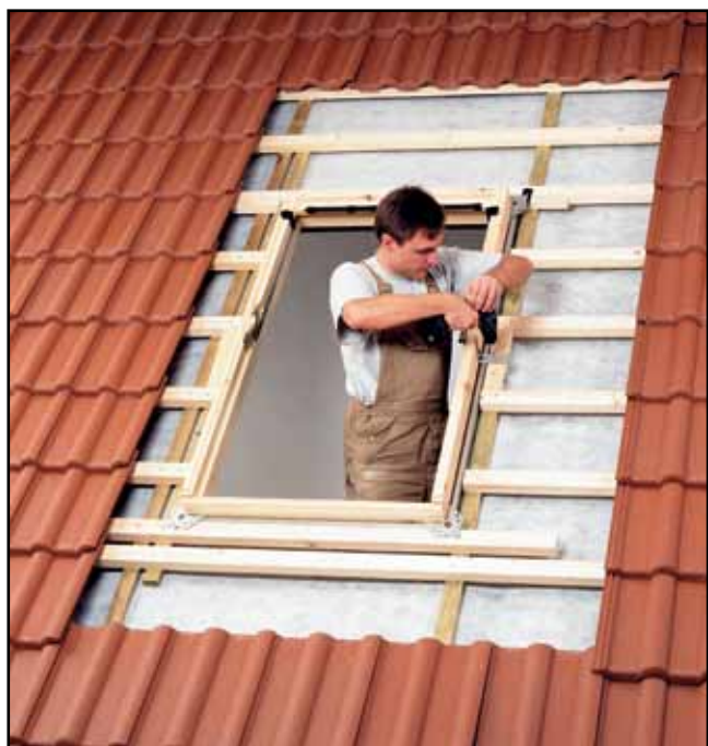
Fig 5.10: Securing the frame
