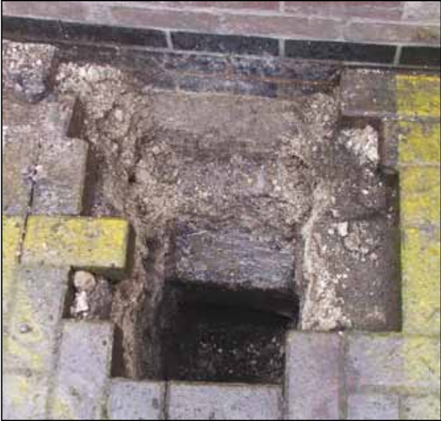
Fig 13.5: Trial hole for foundation inspection
