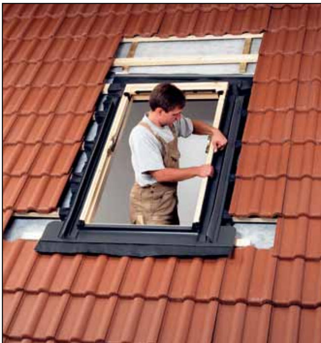
Fig 5.11: Installation of weatherproofing arrangement
