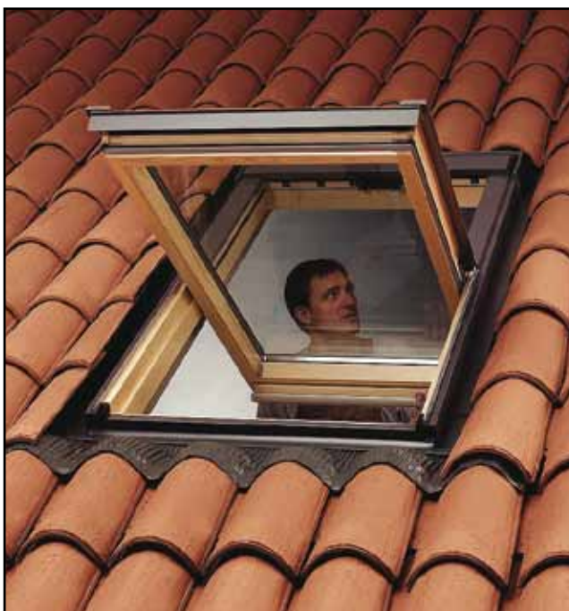
Fig 5.12: The fully installed window
