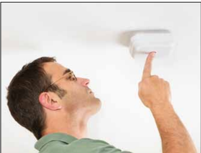
Fig 13.6: Testing smoke alarm
