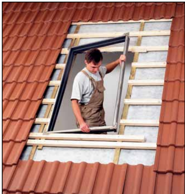
Fig 5.9: Inserting the support frame
