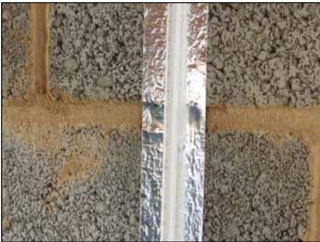
Fig 11.1: Positions for metallic tape by plastic pipes
