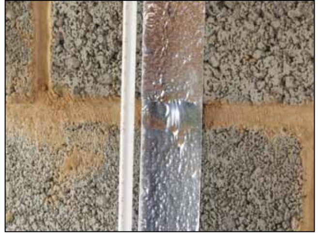
Fig 11.2: Positions for metallic tape by plastic pipes
