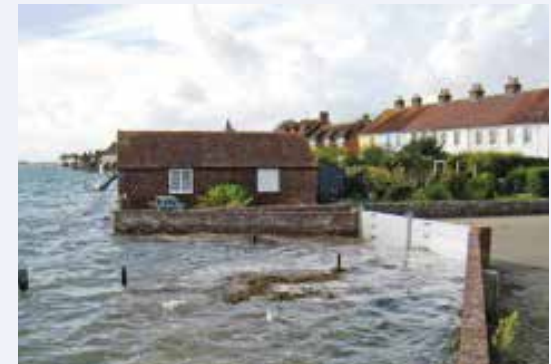
Figure 2 Flood barrier in action
