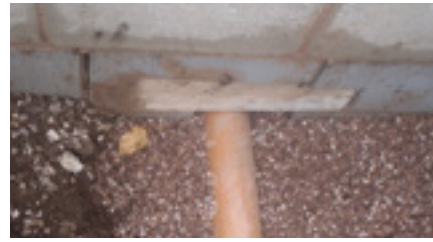
Photo of Lintel over sewer pipe
